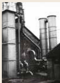
Condensors for removing tar from square tower to scrubber
